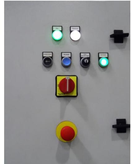
\* The light is on when the Autoblock is in initial position (near the dock) and turns off as soon as it is in action. In case of a vehicle detection option, the light turns on in the presence of a vehicle and turns off when the Autoblock is in action.
